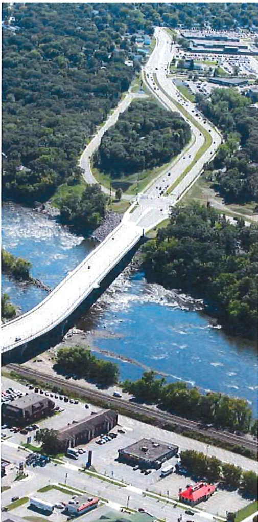
Above: Sauk Rapids Bridge
