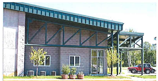
Crow Wing / Crosslake Public Works Facility - 2002
